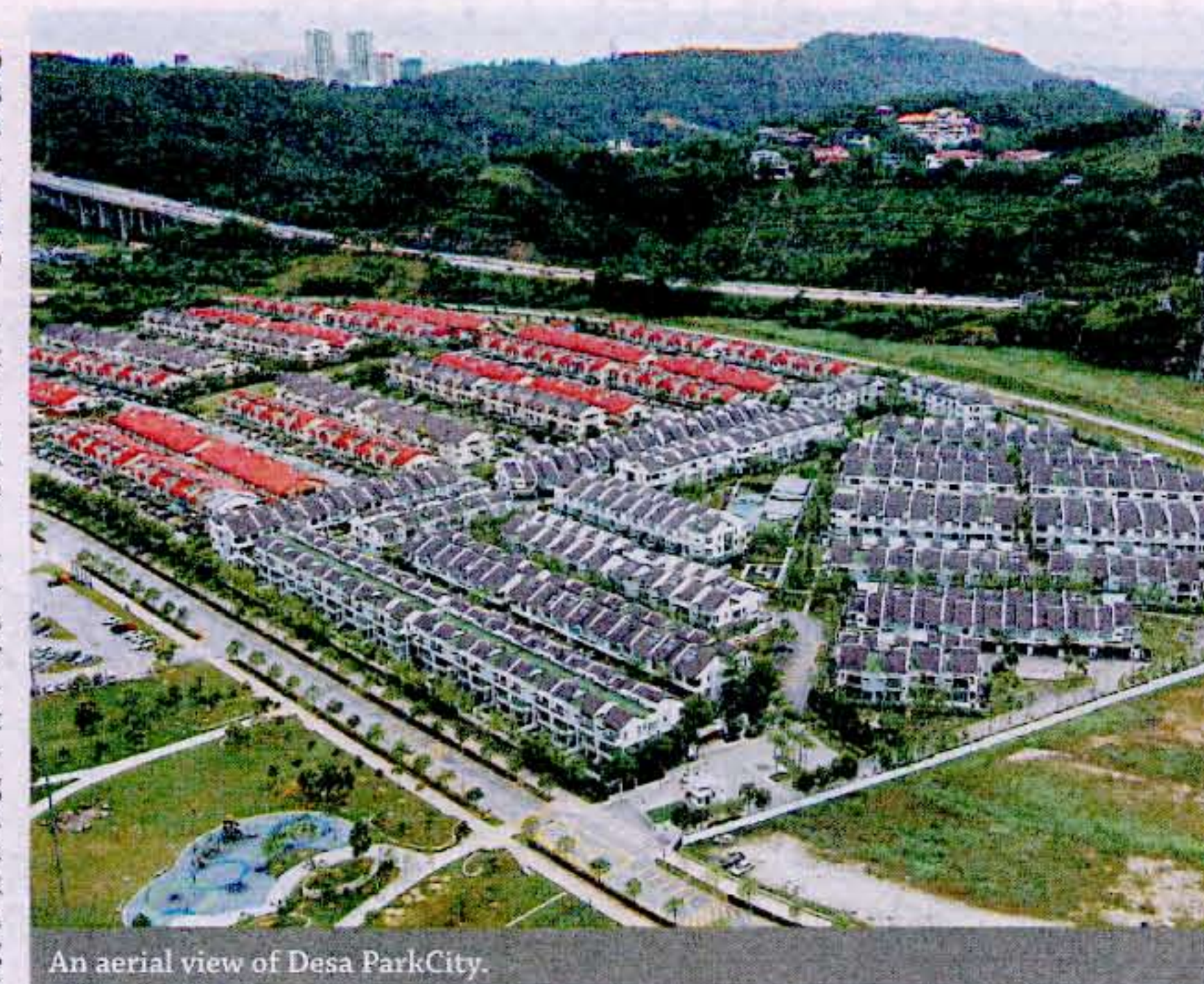
An aerial view of Desa ParkCity.
